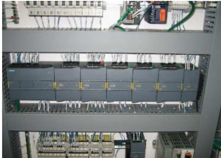
Figure 7: Typical PLC Control
